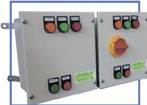
The SAU-PPV (SAU-SPV) fan control cabinet is implemented on the basis of a power disconnector, contactor and thermal electrical relay.
